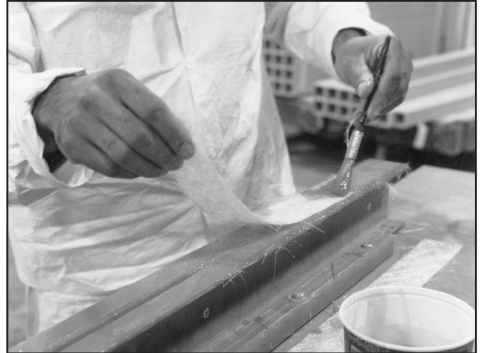
Joint taping with fiberglass mat and polyester resin.
